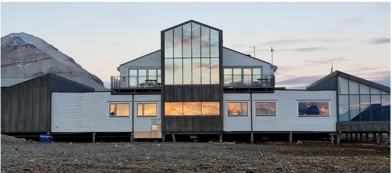
Figure 19. Service building, field BA6 (photo 2022: Dina Brode-Roger, Ny-Ålesund: Visual Profiling)
