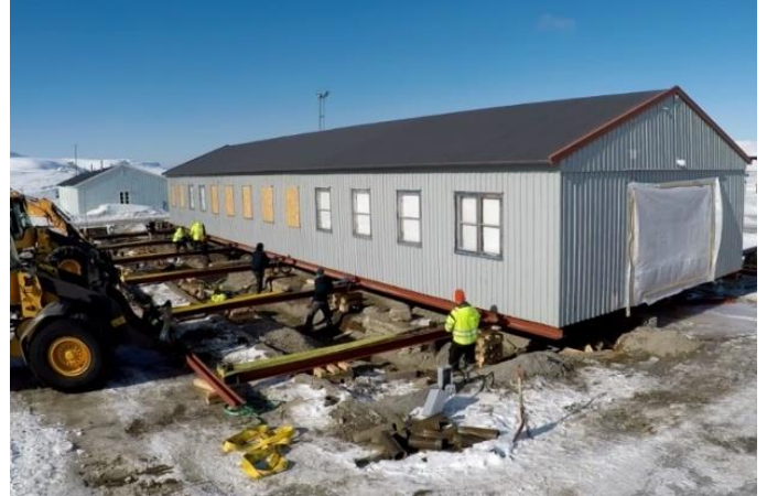
Figure 13. Relaying the hospital's foundations, 2018
