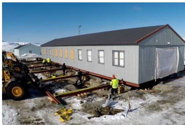
Figure 14. Relaying the hospital's foundations, 2018
