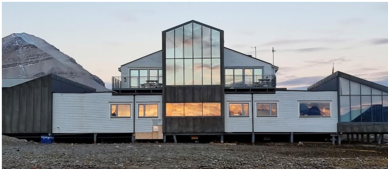
Figure 17. Service building, field BA6
