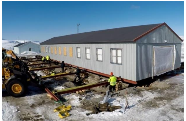
Figur 14. Refundamentering Sykehuset, 2018
